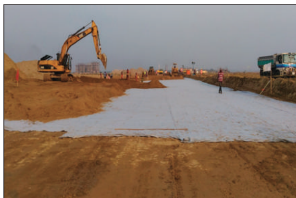
Geotextile Laying Work
