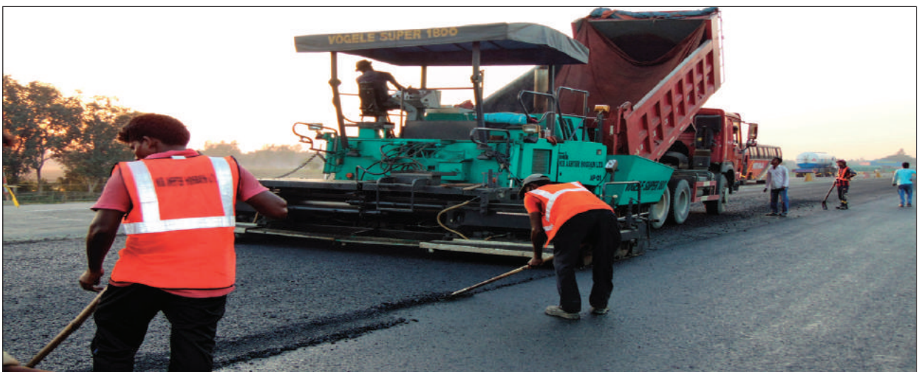
Asphalt Overlay Work on East and West Approach of Bangabandhu Bridge, Tangail & Sirajgonj, 32 Km
