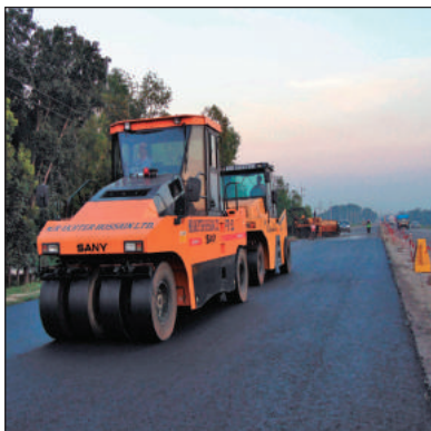
Asphalt Paving Work
