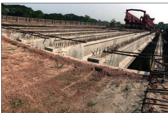
Shifting & Placement of PC Girder Using Launching Girder at Bridge Locations
