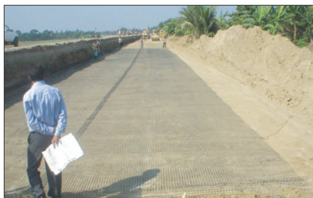
Soil Improvement with Geo-grid
