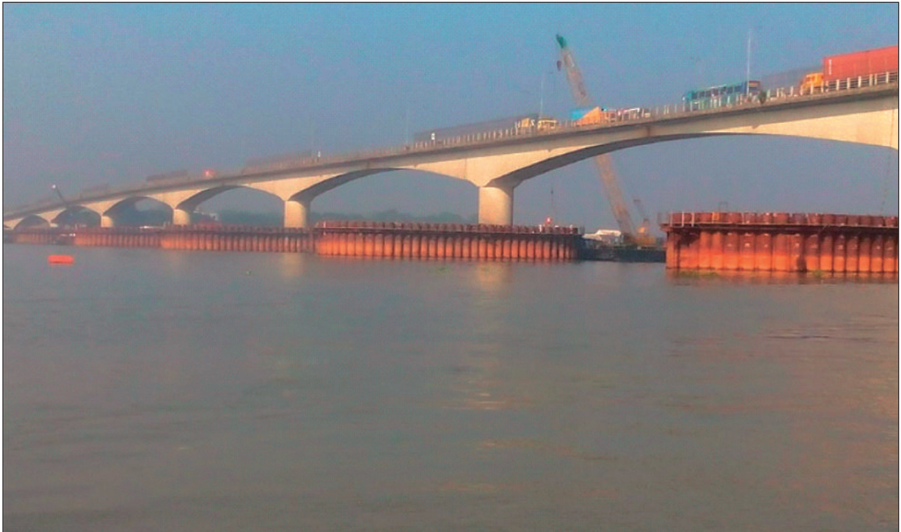
Gumti 2nd Bridge Cofferdam Bridge Pier column under construction
