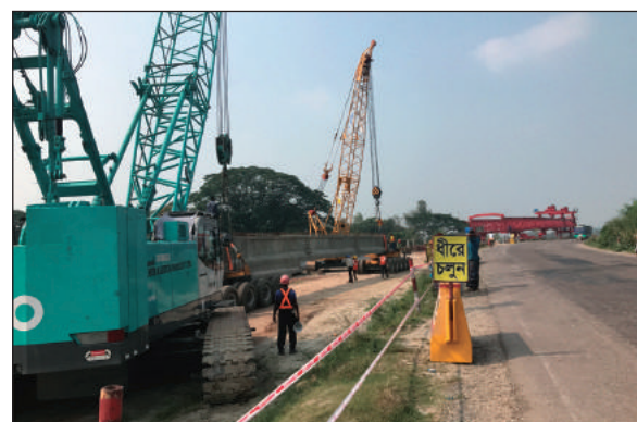
Shifting & Placement of PC Girder Using Launching Girder at Bridge Locations
