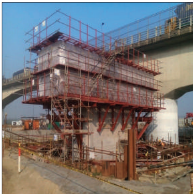
Gumti 2ndBridge_Pier column & Head front side
