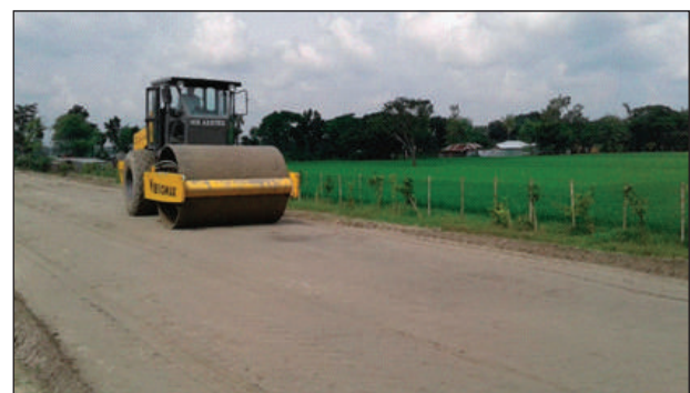
Soil compaction by roller
