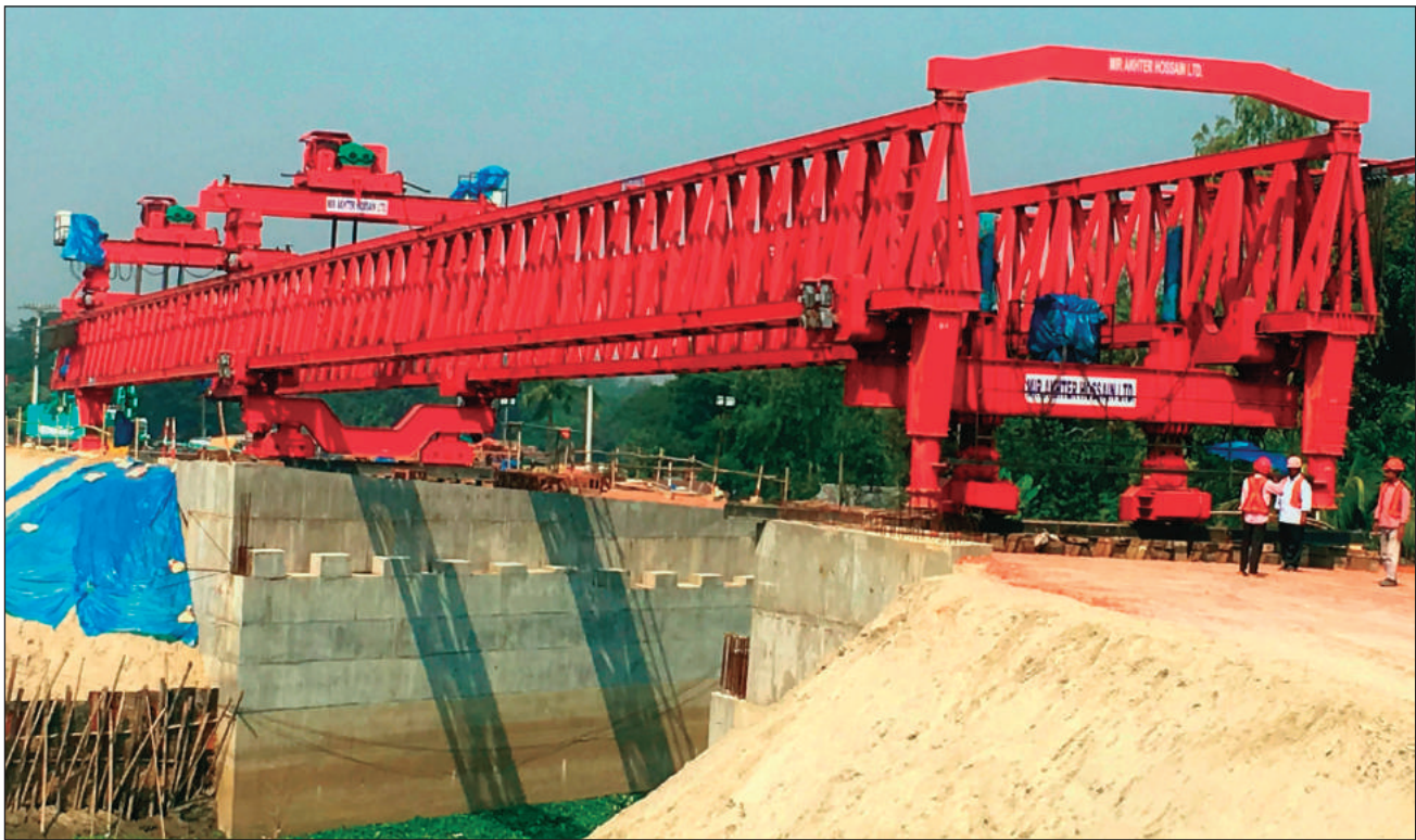
Shifting & Placement of PC Girder Using Launching Girder at Bridge Locations
