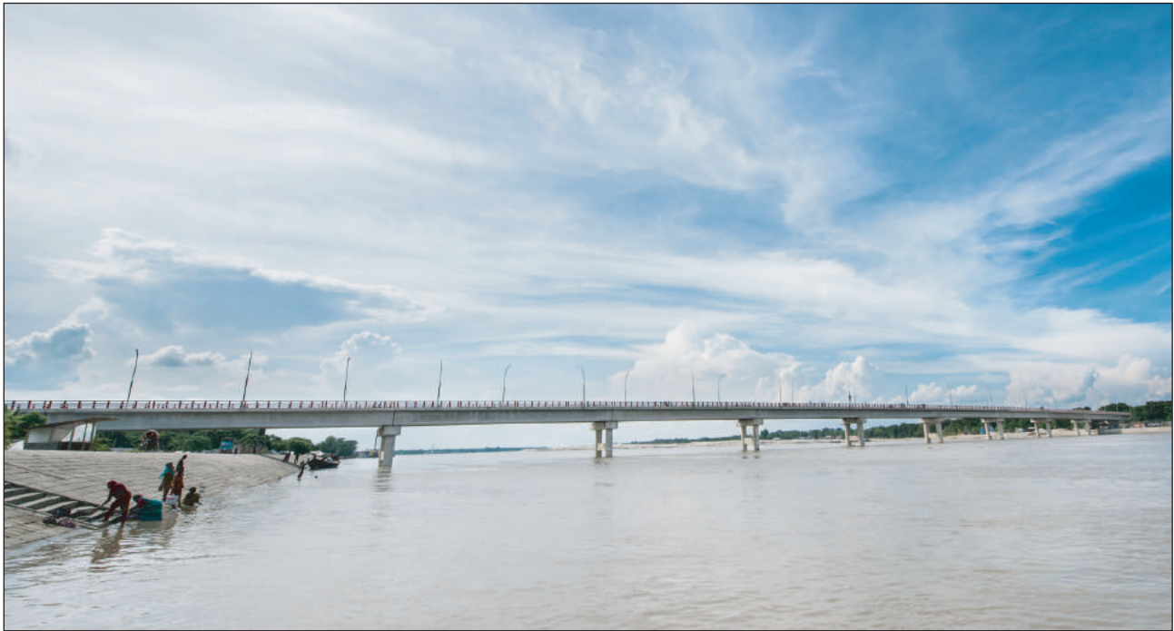
Construction of 604.55m long Pre-Stressed Girder Bridge over Gorai River at Kushtia
