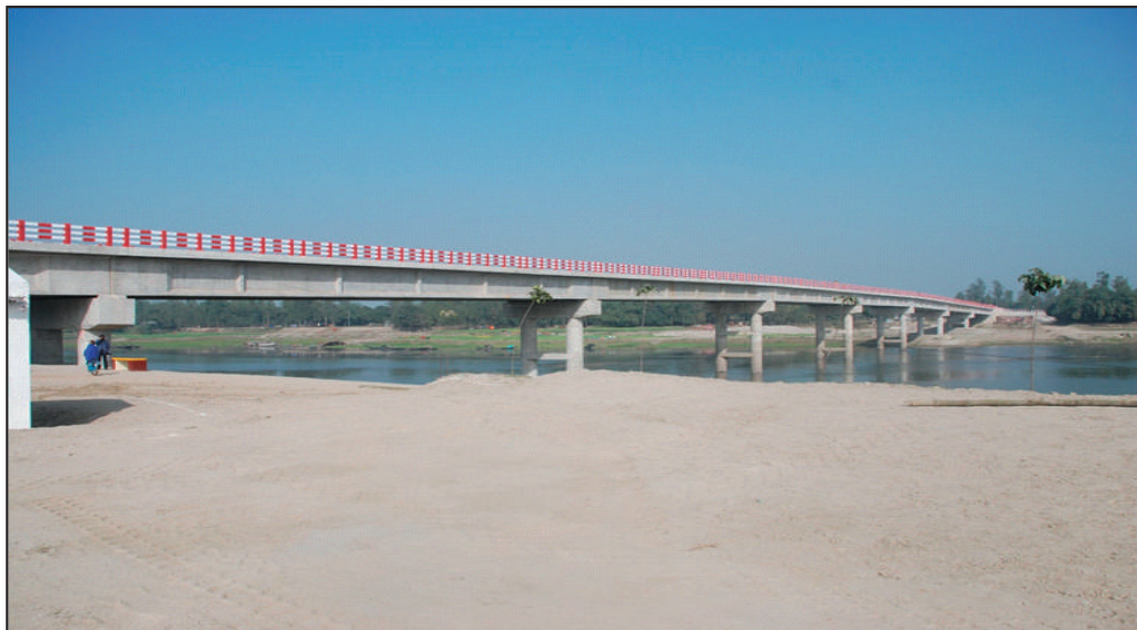
347.295m long PC Girder Bridge over Karatoa River at Sontola Ghat on Ullahpara Belkuchi Road
