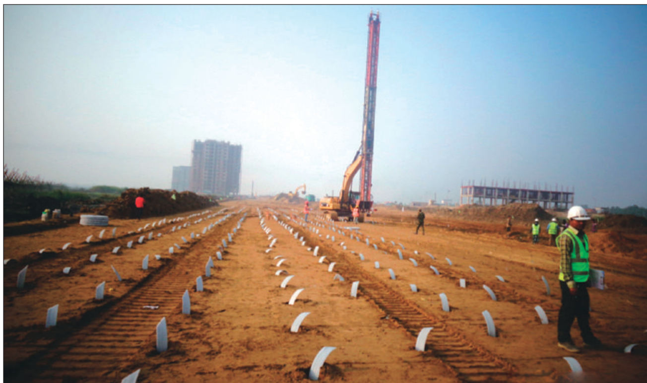
62 Prefabricated Vertical Drain (PVD) work in progress
