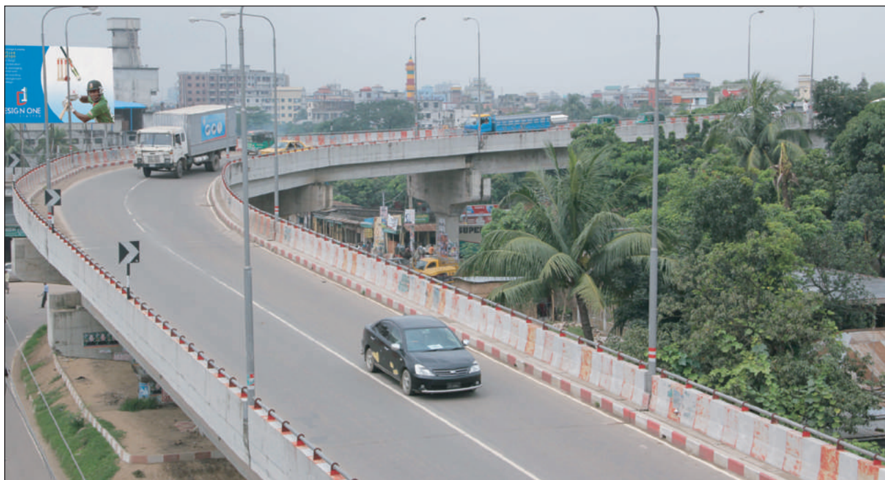
566m long Flyover including Approach Road with Nehemiah Anchored Earth retaining Wall
