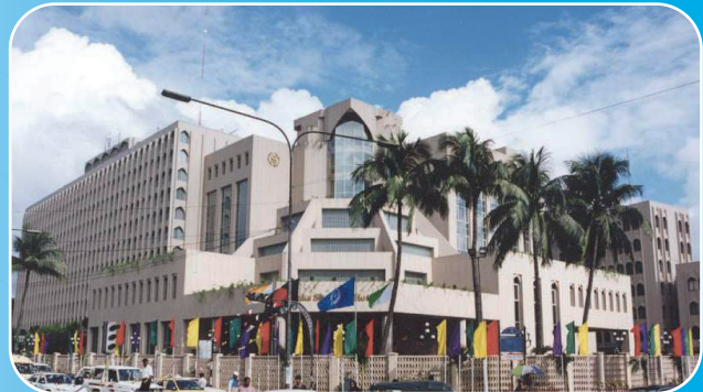
Project Name: New Block of Dhaka Sheraton Hotel
