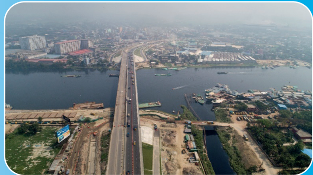
Project Name: The Construction of Kanchpur, Meghna and Gumti 2nd Bridges And Rehabilitation Of Existing Bridges (Pw-01)
