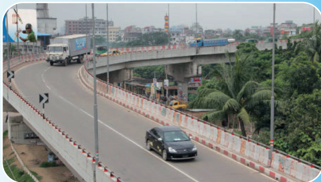
Project Name: Tongi Flyover with Nehemiah Anchored Earth Wall
