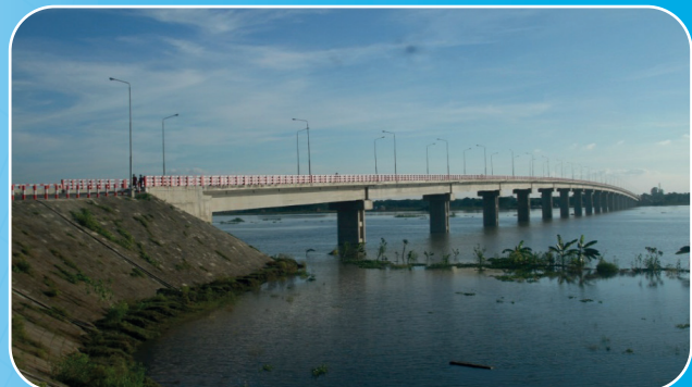
Project Name: Construction of 810m Long PC Box Girder Bridge on Saltia Bazar-Hazigonj Bazar-Dewangonj Bazar Road over the old Brahmaputra River
