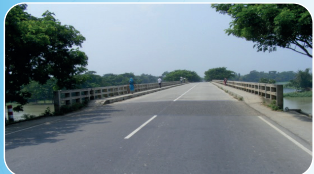
Project Name: Construction, Replacement of Reconstruction of Bridge at Seventeen (17) Location in Dhaka Zone through Contract Package No. EBBIP/ Dhaka/CP-01 under Eastern Bangladesh Bridge Improvement Project
