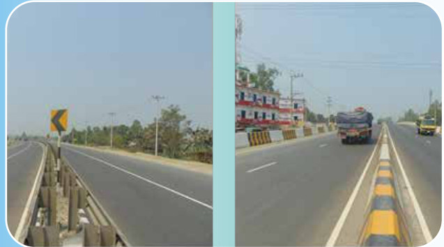
Project Name: Construction of SASEC 4-LANE ROAD PROJECT, CONTRACT NO-3, DULLAMARI ROAD TO TANGAIL (22.4 KM)
