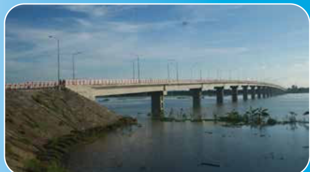
Project Name: Construction of 810m Long PC Box Girder Bridge on Saltia Bazar-Hazigonj Bazar-Dewangonj Bazar Road over the old Brahmaputra River
